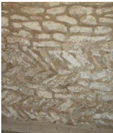
Fig. 2a Internal herringbone masonry, north tower wall.
