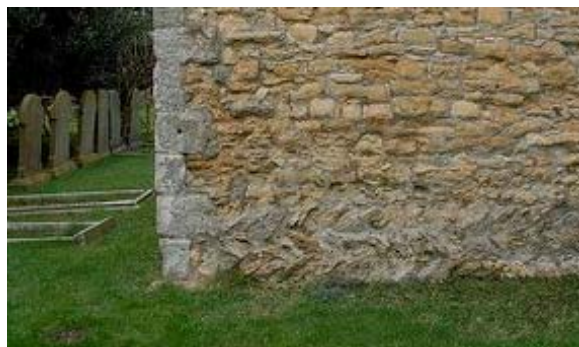
Fig. 2b External herringbone masonry, south tower wall
