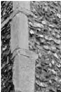
Fig.5 Saxon long-and-short work
